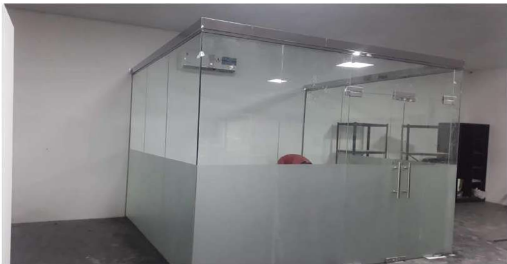
Fit Out Work
